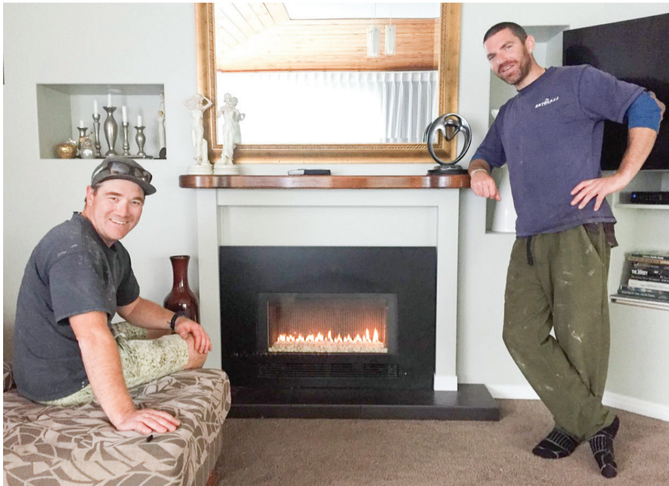
Ben Gibson and James Scott installing a fireplace.
